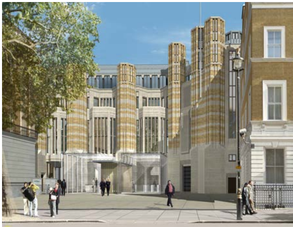
Images by JjGallery for Jonathan Louth Architects
