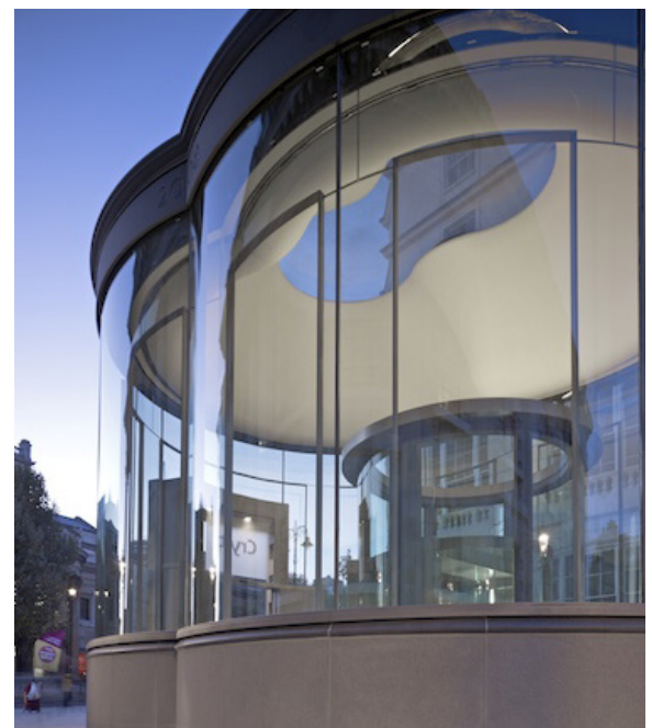
St Martin-in-the-Fields - Nigel Lea whilst at Eric Parry Architects. Won RIBA London & Design for London Public Space Award, RIBA London & English Heritage Award for Sustaining the Historic Environment
