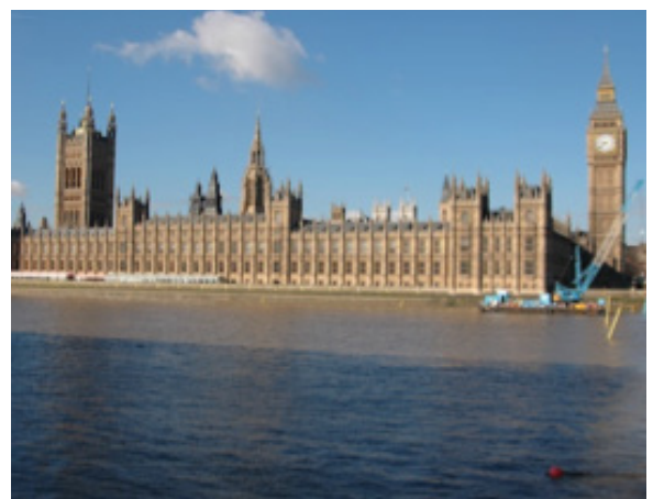
Palace of Westminster, Infrastructure Rationalisation, Repair and Replacement Project - Delivered by Trevor Butler
