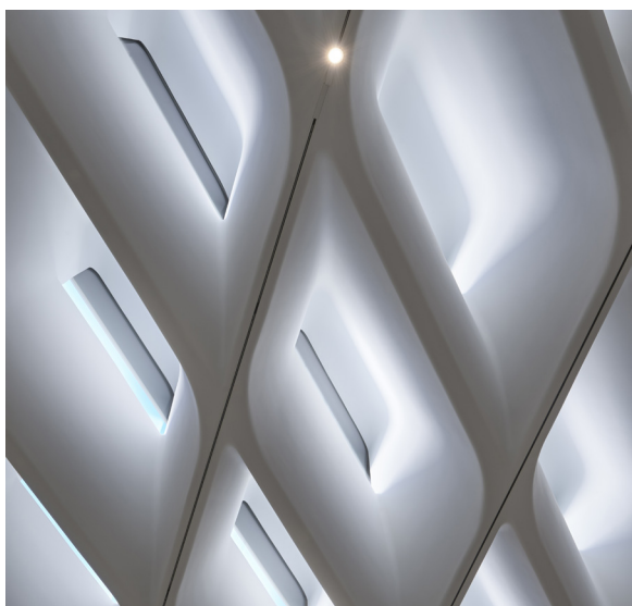
Detail of the 'veil' facade cladding
