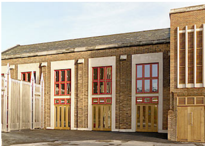
Left: Remodelled facade of Amigo Hall with new elevated lift shaft, stone work derived from the Bapistry, and Jonathan Louth Architect's stainless steel 'Archbishop's Gates'
